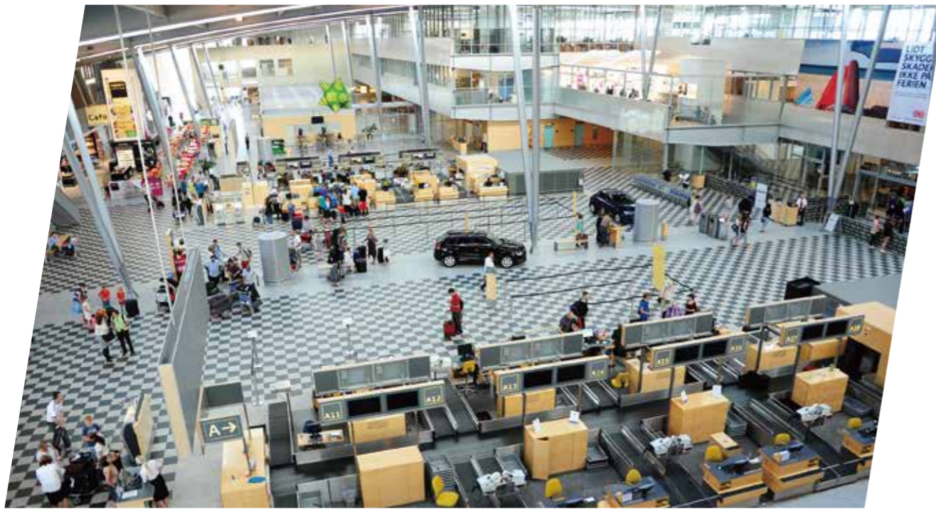
INSTALLED PRODUCTS: VXC SERIES (VA version)
